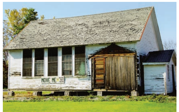
Coonsville Schoolhouse as it stands now at the Manchester Transfer Station
